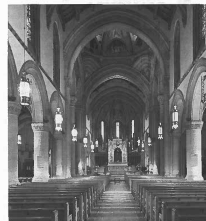
St. Bernard's has a true Gothic vault, where the ribs of stone make a cage to provide a base for the roof. The massive interior is beautified by frescoes and carvings on the walls and ceiling, and the pan-tiled roof has gargoyles.
